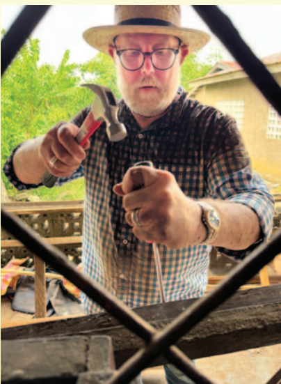
Lt. Scott Smith repairs a windowpane at the Yenge Social Institute.
